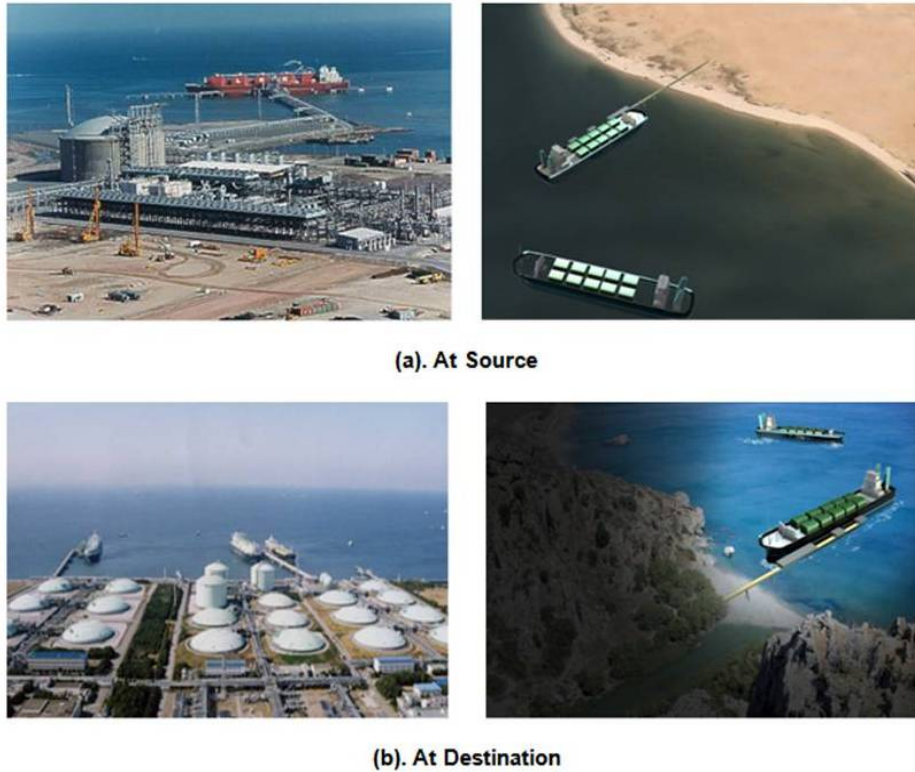
Figure 1 Loading and Offloading Terminal for LNG and CNG (Source: XGAS website http://www.xgas.us )
