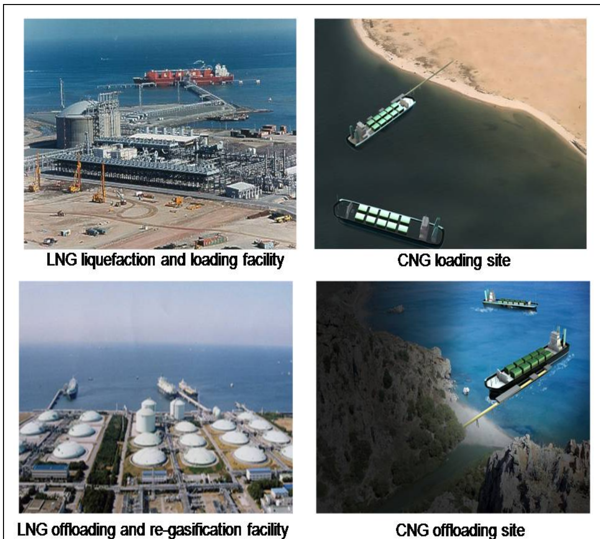
Figure 4: Loading and offloading facilities for LNG and CNG, from XGAS, 2008.
